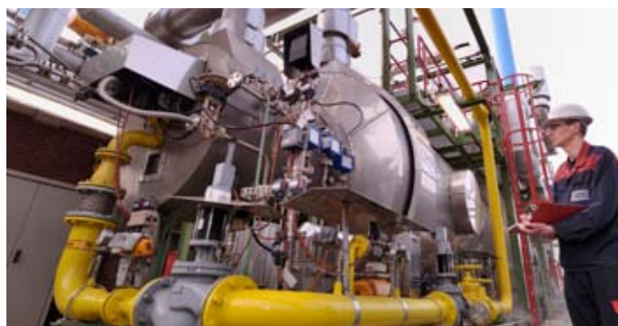
The reduction plant separates nitrous oxide into its constituents – oxygen and nitrogen – at high temperatures. The heat created generates steam that is fed into the supply network at the Krefeld-Uerdingen CHEMPARK site for further use.
